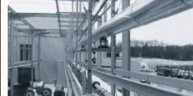
CV-Rohre in wetterfester Ausführung | CV tubes of weather-proof design
